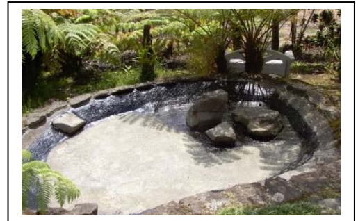
Perimeter coated with Liquid Rubber
